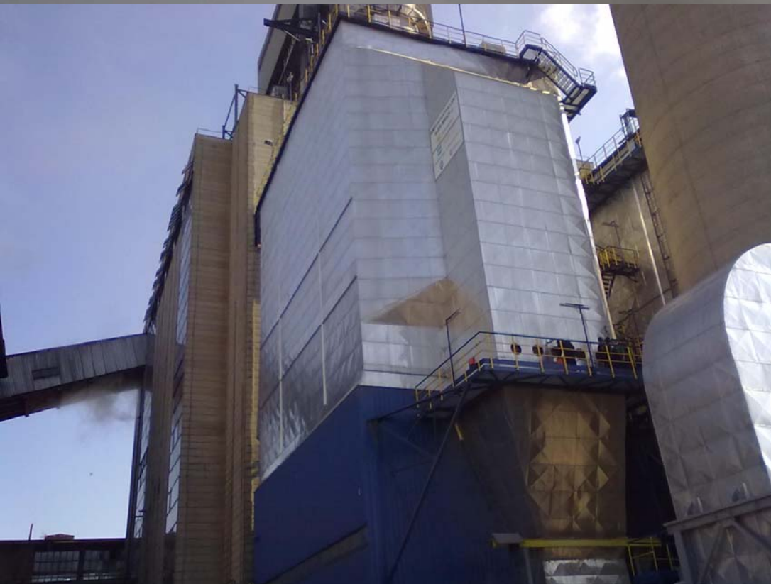
Figure 2. Right electrostatic precipitator – rear view
